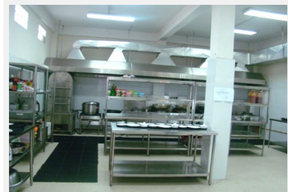
INSTALASI GIZI | NUTRIENT INST
